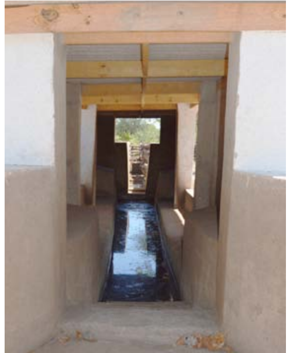
The newly constructed Kasibo cattle dip tank.
