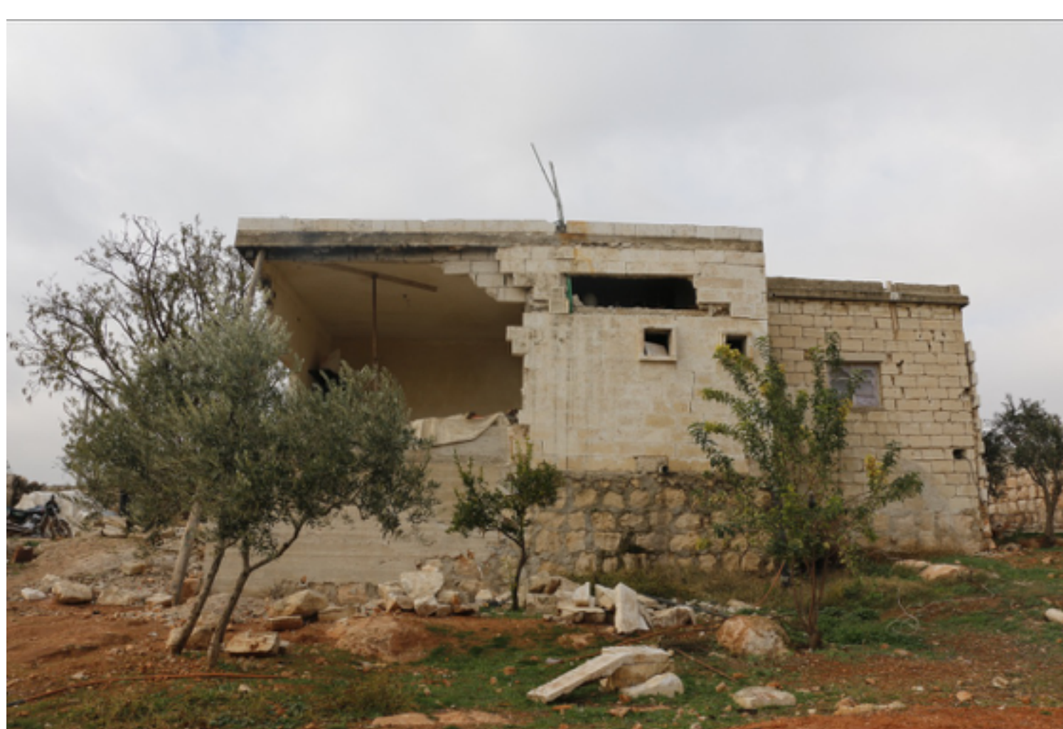
House of Nader, hardly damaged by shelling.
